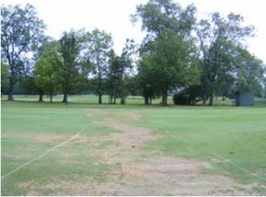
Inadequate Fairway Drainage
